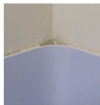
Gap between skirting and walls
