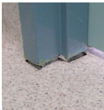
Figure 28: Gaps between door frame and floor
